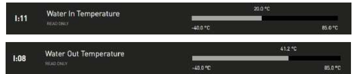
Water temperature control
