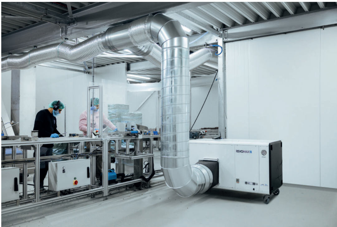
RevomaxII sep-fan and custom aluminium airhoses. The fan is installed integrated in the airhoses.
